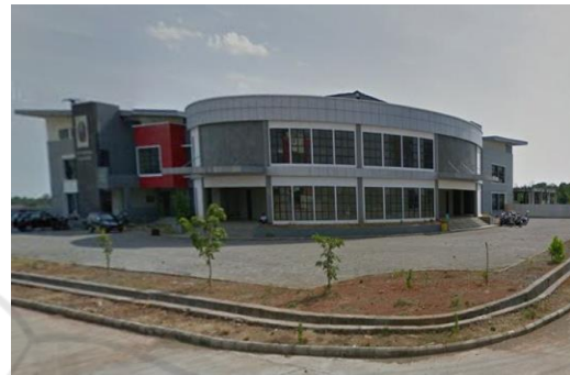
Figure 2: Electrical department building from left side.
