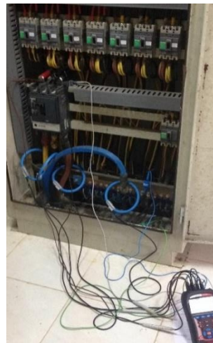
Figure 5: Installation of combined power measurement.
