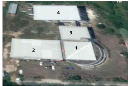
Figure 1: Buildings of Electrical Engineering Dept.
